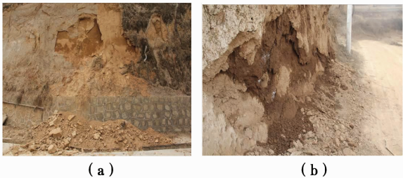
图 1 黄土边坡冻融剥落病害 Fig.1 loess slope spalling hazards under freezing-thawing cycles
