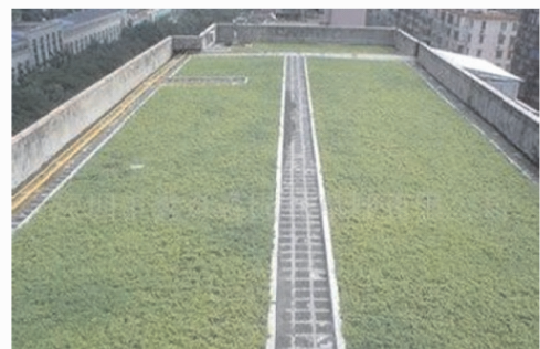
Fig. 1 LEG roof applied in this case
