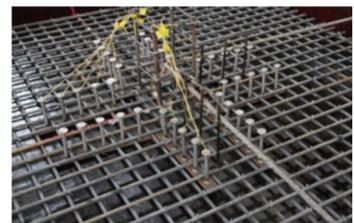
图9 栓钉测点布置
