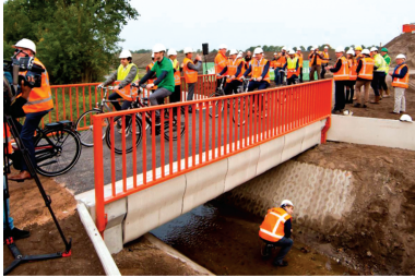
图 5 3D 打印混凝土桥 [83]
