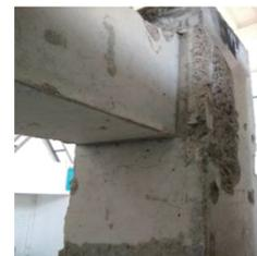
(c) Micro-cracks and concrete burst
