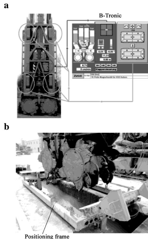
Fig. 8 The precision control of trenching: a) inclinometer system [20], b) positioning frame
