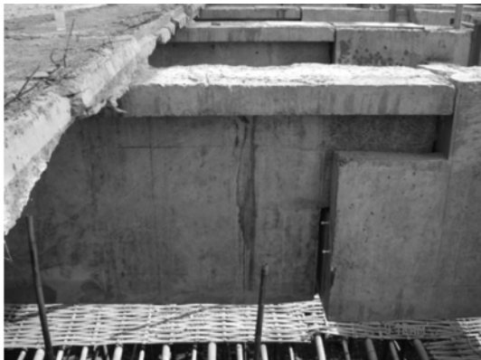
Fig. 2 Corbels of the Dangtu Road Bridge before reinforcement
