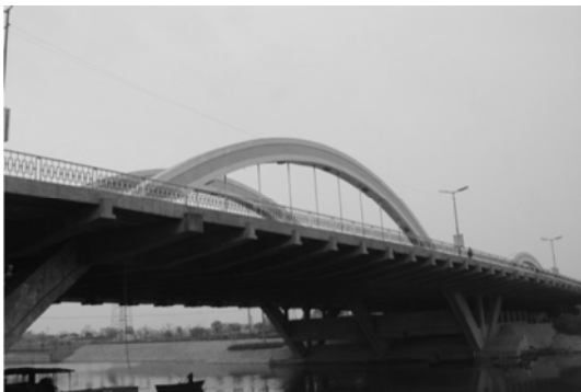
Fig. 1 The Dangtu Road Bridge in 2007
