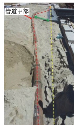
图 7 “滑坡/断层”试验结果示意图 [44] Fig. 7 Schematic diagram of landslide/fault test results [44]
