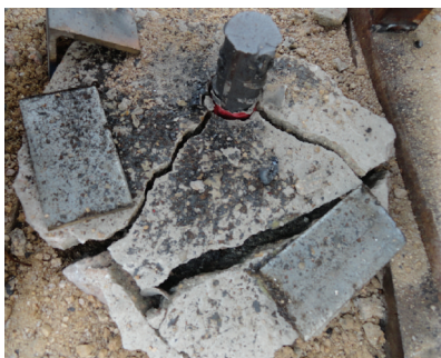
(a) 锚筋拔断
