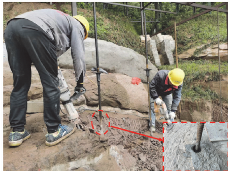
(a) 锚杆灌浆
